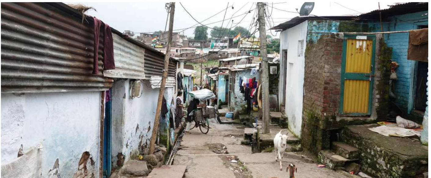
Figure 5 - Condition of the existing slum in the prohibited zone.
