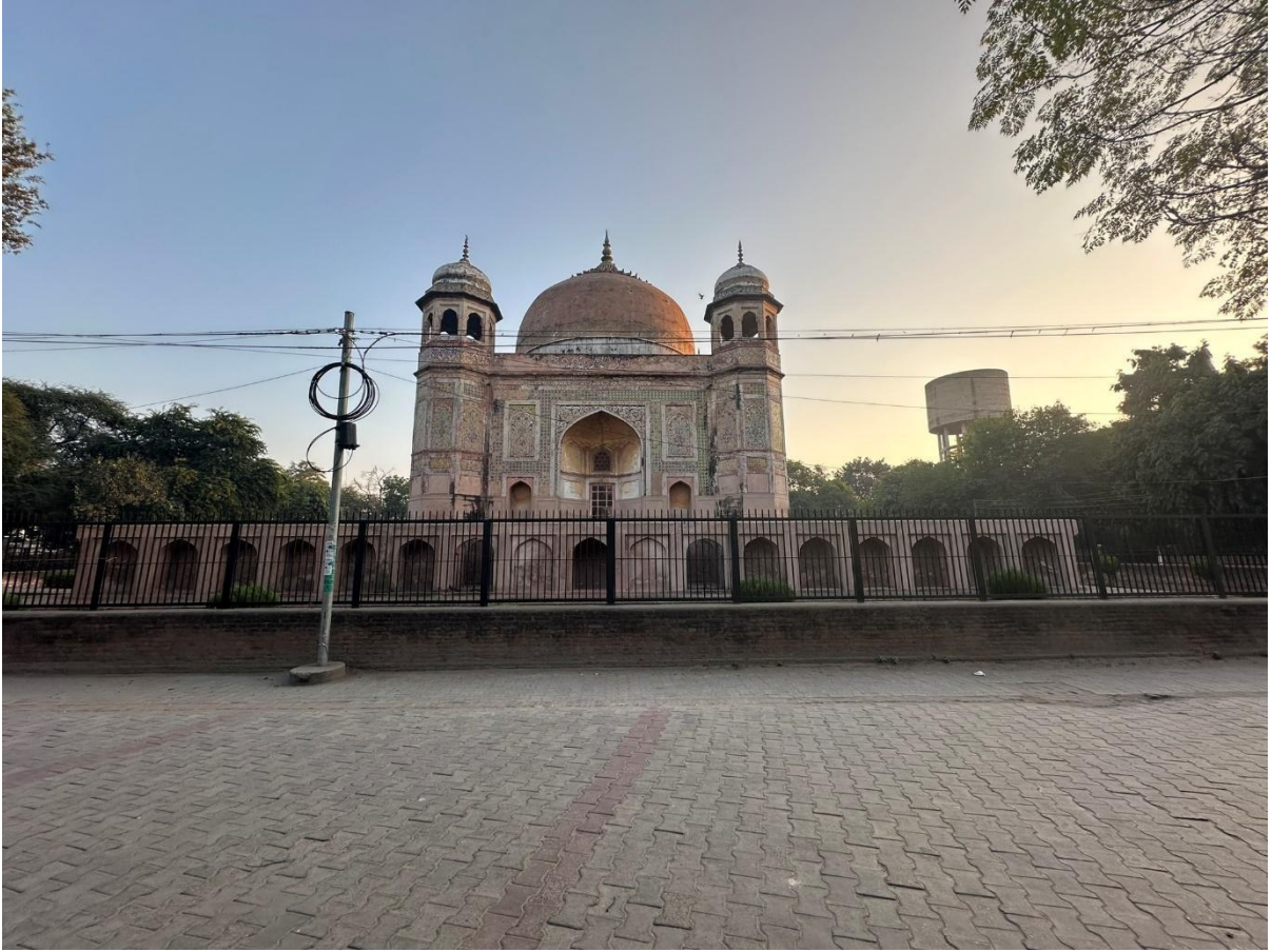
Figure 6.9: View of the monument from the western direction of the prohibited area.
