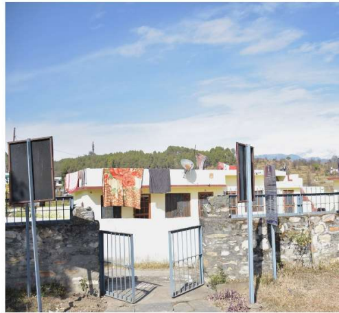
Image 11: View of the newly constructed house in front of the entrance gate.
