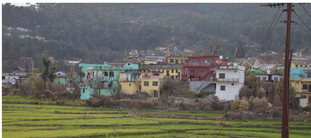
Image 49: Newly constructed double and triple storey houses along the periphery of the village with the shikharas of Rakshas Deval temple and Lakshmi Narayan temple visible in the backdrop.
