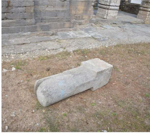
Image 17: Stone shaft fallen from top of the shikhar.
