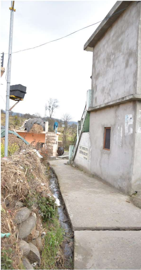
Image 44: Storm water drains laid in the village.
