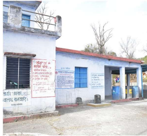
Image 39: Panchayat Ghar with some sculptures kept in the open space.
