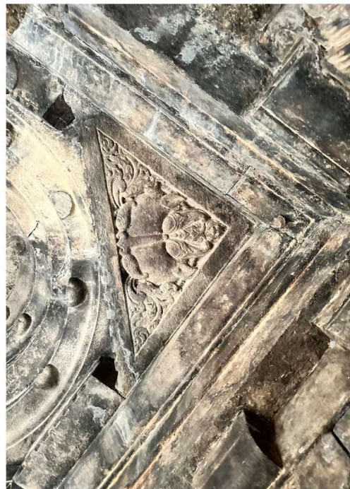
Image 31: Carving of a kirtimukha on the corner slab of the ceiling of the mandapa.
