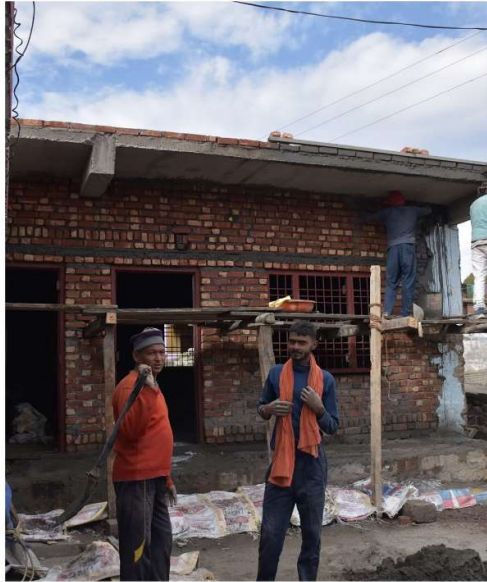
Image 22: An under-construction house in close proximity to Lakshmi Narayan Temple.
