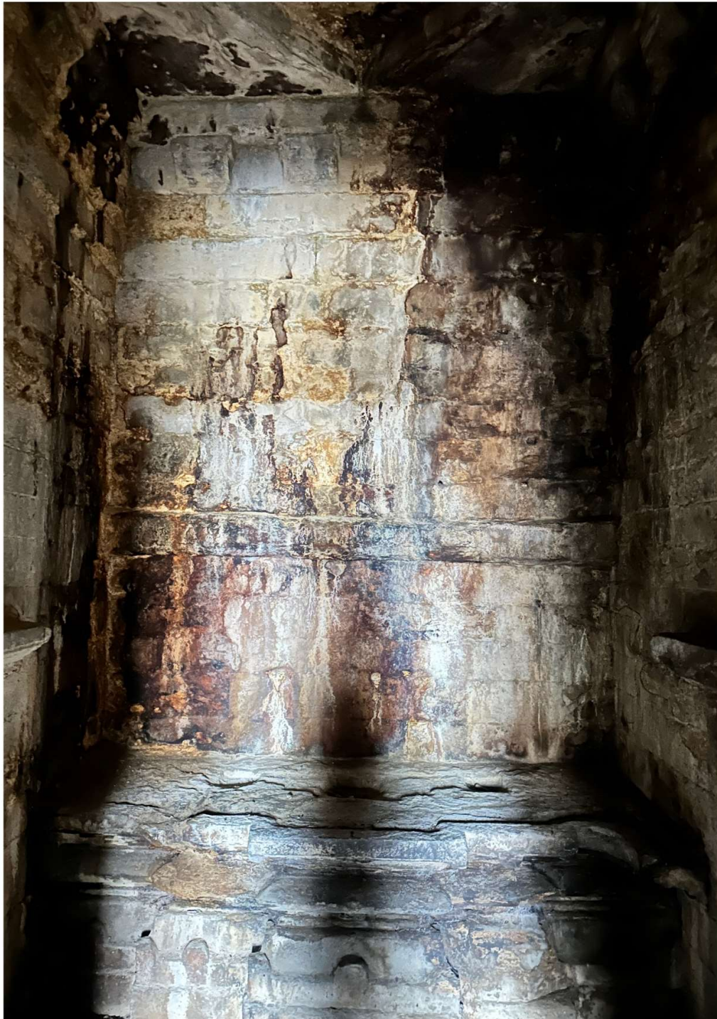
Image 32: Deteriorated condition of the garbhagriha due to prolonged water seepage.
