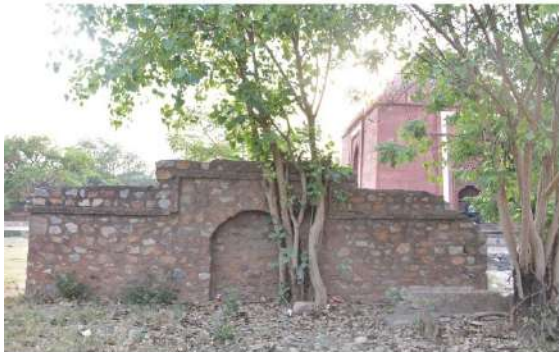
Image 08: Ruined structure on south side of Gateway.
