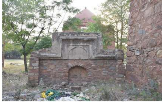
Image 07: Wall Mosque located on south side of Gateway.
