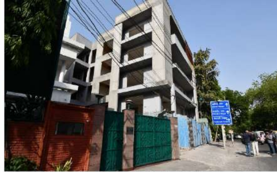
Image 30: Under Construction Plot inside Regulated area.
