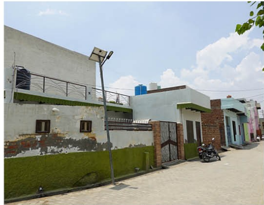
Image 10- Recently built Residencies in the Prohibited area on western side.
