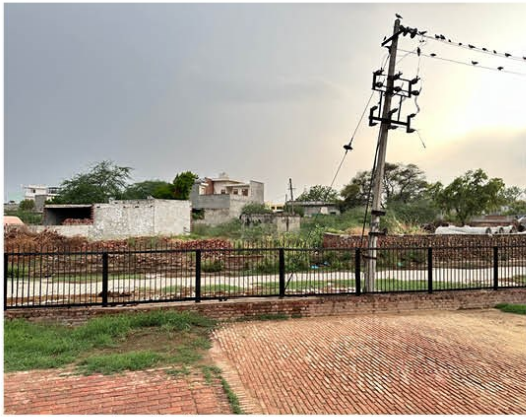
Image 14- Residential buildings in the close proximity of baoli on western side.
