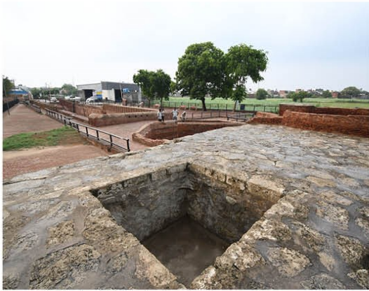
Image 25- Missing of Railing in the well.
